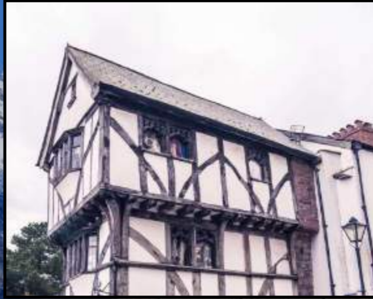
Timber laced masonry
