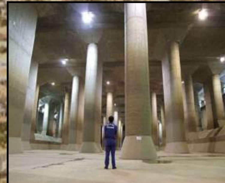
Underground Flood channels
