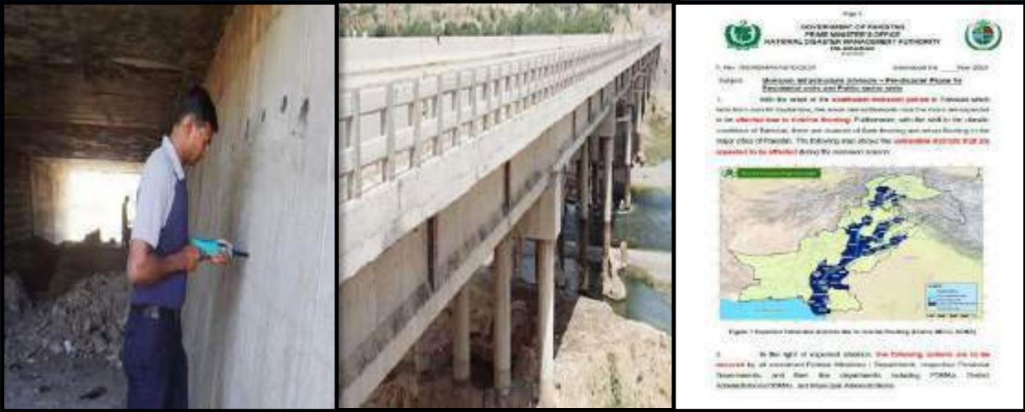
Audit / monitoring of existing Infrastructure
