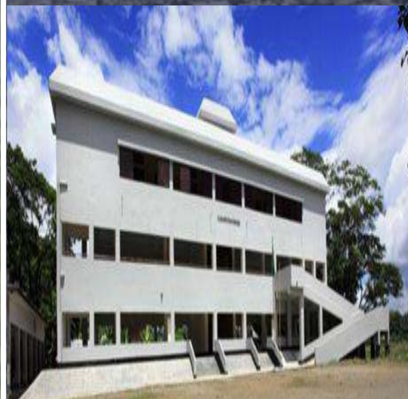
Use of Modern Construction Tech
