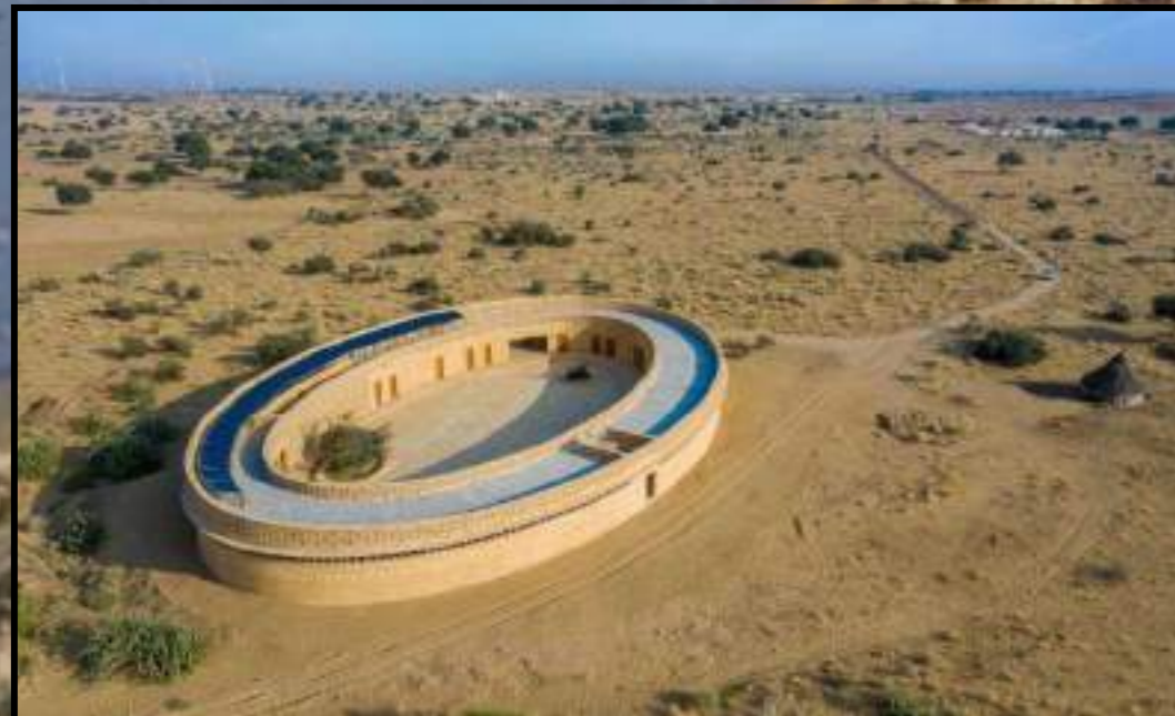
Solar Panels installed, Constructed by local craftsmen
