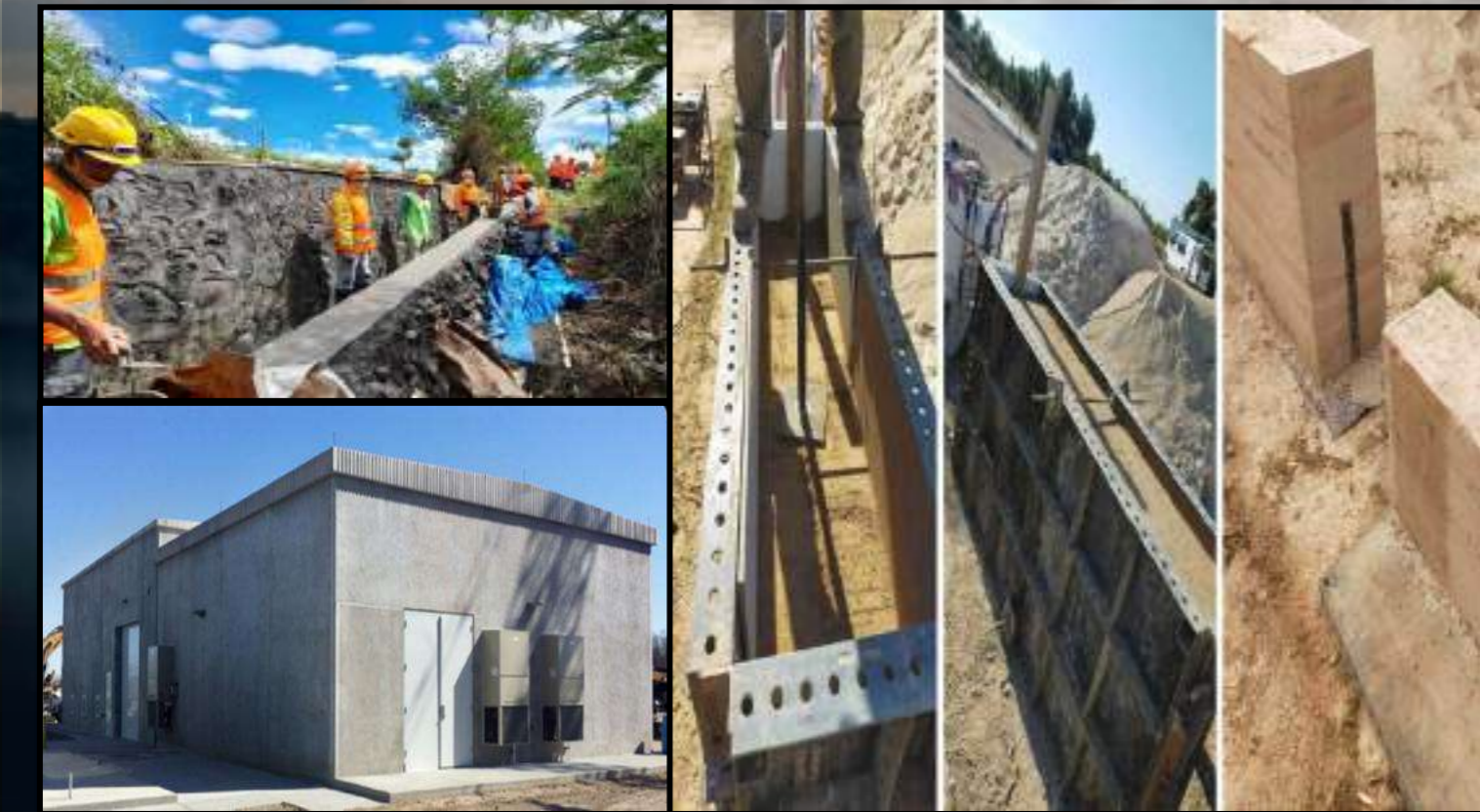
Course corrections measures for new construction
