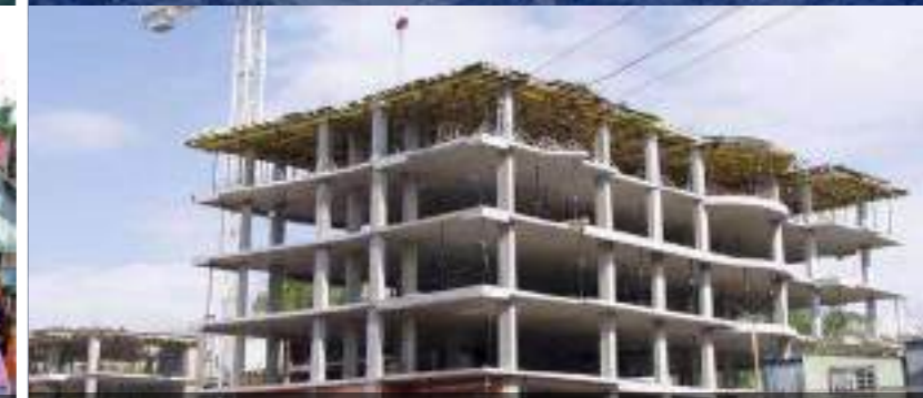
Moment Resisting Frame RCC
