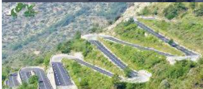
Slope Stabilized Roads
